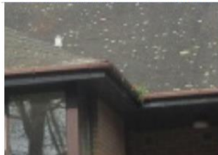
Vegetation should be removed from gutters ensuring free disposal of rainwater
